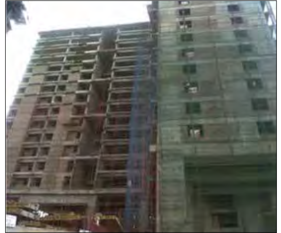
Tower Middle and West
